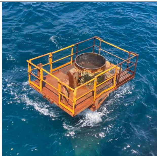
Existing pile cut for new top section
