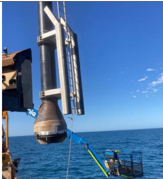
Lifting new top section into position
